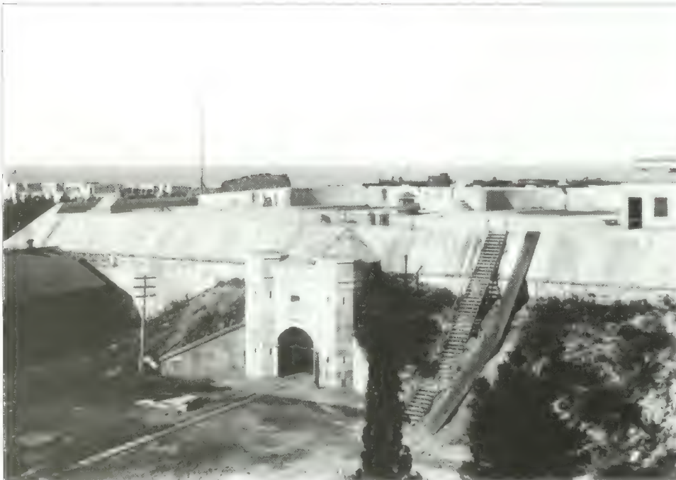
Figure 2.27. View looking northeast at Battery Potter, circa 1906. Between 1901 and 1903, the Army constructed a central powerhouse and coal shed for Fort Hancock's lighting system near the northwest corner of Battery Potter. A portion of engineered earthwork on the battery's west facade was removed to accommodate the buildings, visible on the left (GATE 7818).
